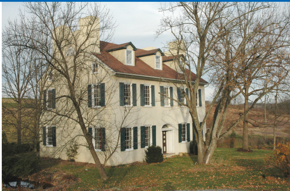
BEFORE AND AFTER: Valley REC member Jean Murphy spent 20 years refurbishing the 1800s Christian Oyer Jr. House in Huntingdon County. Her efforts have provided her a beautiful home and placed the property on the National Park Service Register of Historic Places. The undated photo, below left, shows the house at its worst. Notice the dormers are missing. (Photos by Doug Roles)
