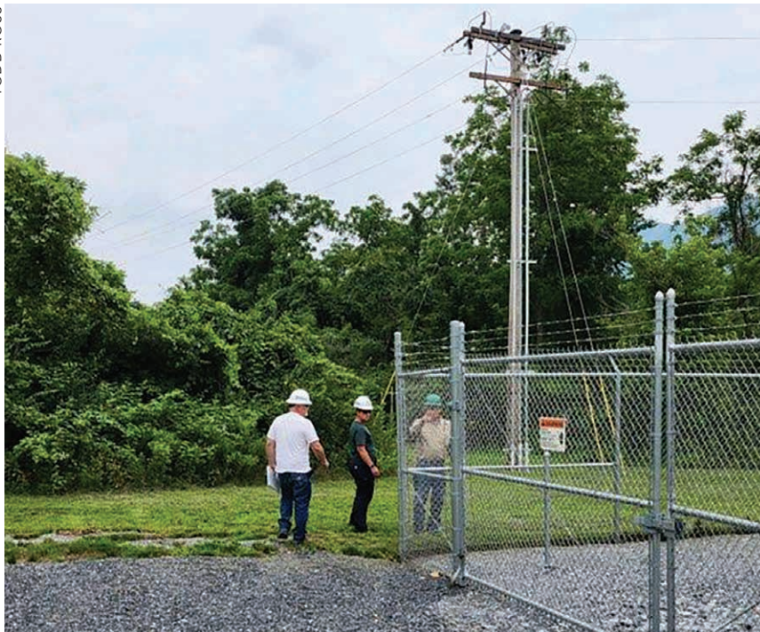
SUBSTATION INSPECTION: From left, Mike Chamberlin and Heather Holt from Gettysburg-based Adams Electric Cooperative inspect the fence around the Path Valley substation with Joe Selnekovic, manager, Job Training & Safety/environmental adviser at the Pennsylvania Rural Electric Association.
